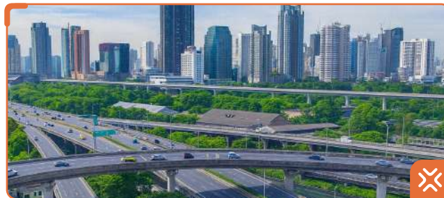
Infrastructure Works, NOIDA | UP
