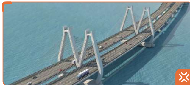
Versova Bandra Sealink | MH 1DPMS for 8 Lane Versova Bandra Sealink of 17 KM | ₹ 6900 Cr.
