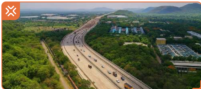
DPMS of 8 Laninig of NH-848 (Vadpe Thane Section) | MH 8 Lane (MC) & 4 Lane (SR) of 20 KM & 2 Creek bridges. | ₹ 1182 Cr.
