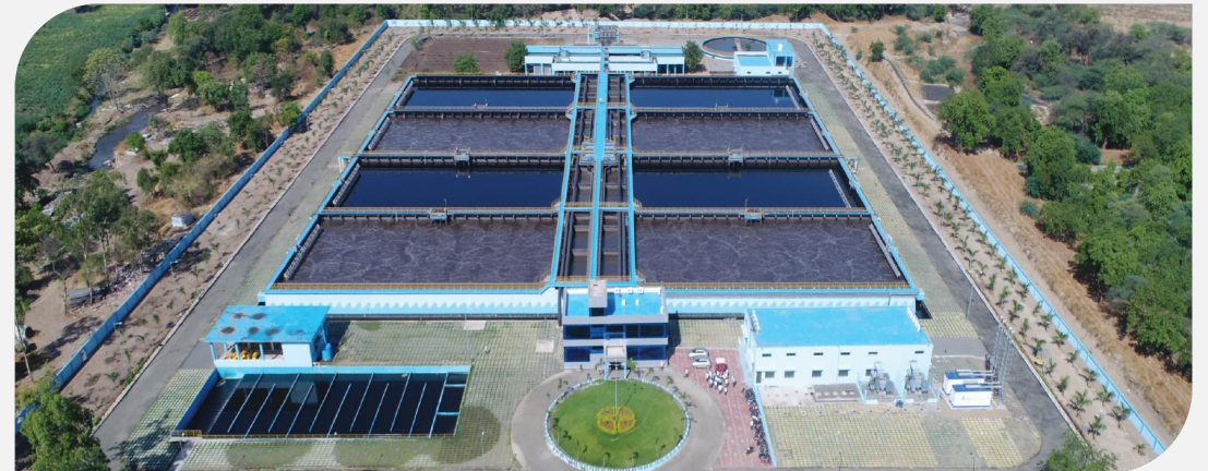
Ch. Sambhaji Nagar Sewerage Scheme, Maharashtra Integrated Underground Sewerage System for 2 Mn population with 603 km of collection network, SPS, 216 MLD STP, & SCADA | Rs. 470 Cr
