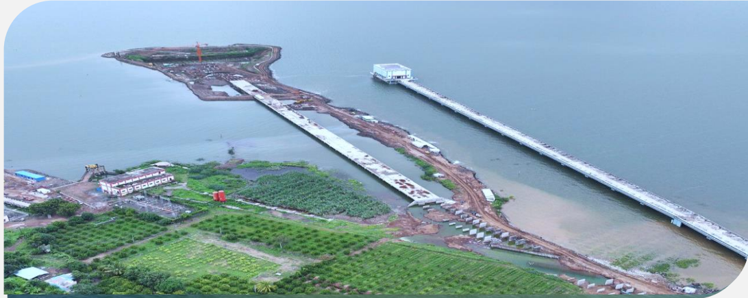
Ch. Sambhaji Nagar Water Supply Scheme, Maharashtra 24x7 Water Supply Scheme for 2 Mn population with 1900 Km Distribution & 78 Km Rising Main, 392 MLD WTP, 2 MBR, 49 ESR & 4 GSR with 104 million CuM capacity | Rs. 2750 Cr
