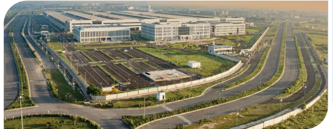
Integrated Industrial Township, Greater NOIDA, Uttar Pradesh Integrated infrastructure for greenfield industrial township over 302 Ha at Greater NOIDA | USD 51 Mn
